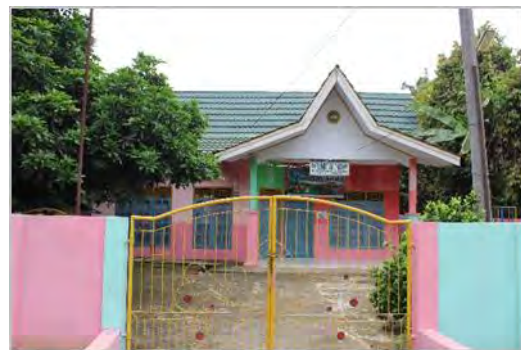
Figure 16 – Kindergarten in Gurun Mudo. Photo taken by the author (2017).
